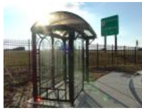
The new Leesburg bus shelter is designed to keep waiting passengers dry and comfortable.
